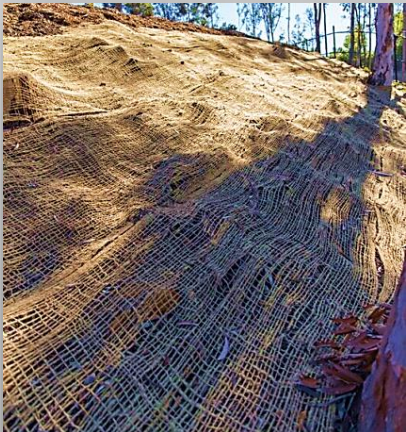
Stabilize eroding slopes
