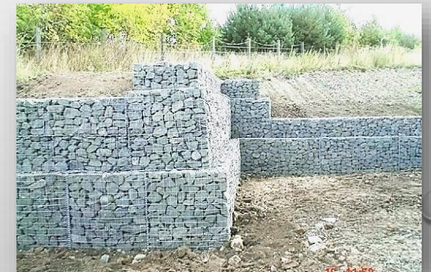
✓ Using riprap or gabions to slow and dissipate stormwater flows
