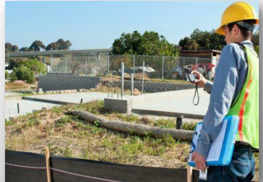
Inspection of sediment control BMPs
