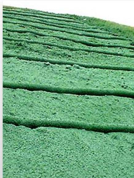
✓ Applying hydro-mulch
