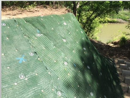
✓ Using geotextiles or mats on slopes
