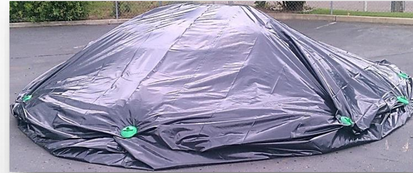
✓ Using plastic tarps to contain stockpiles
